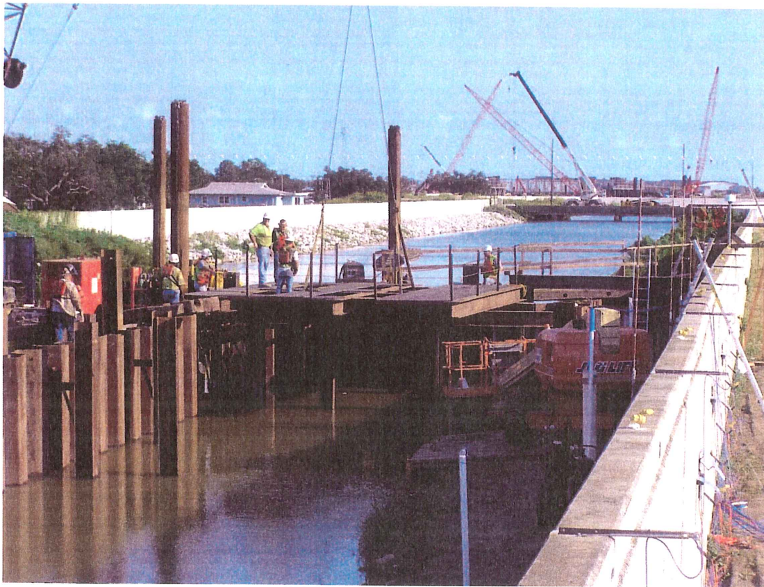
Figure 2.7 – View of Partially Completed Cofferdam (Looking north)
