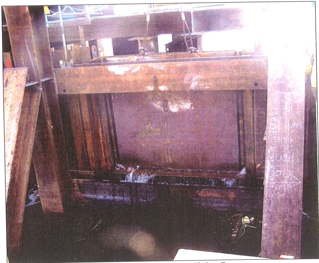
Figure 2.11 – Emergency Sluice Gate
