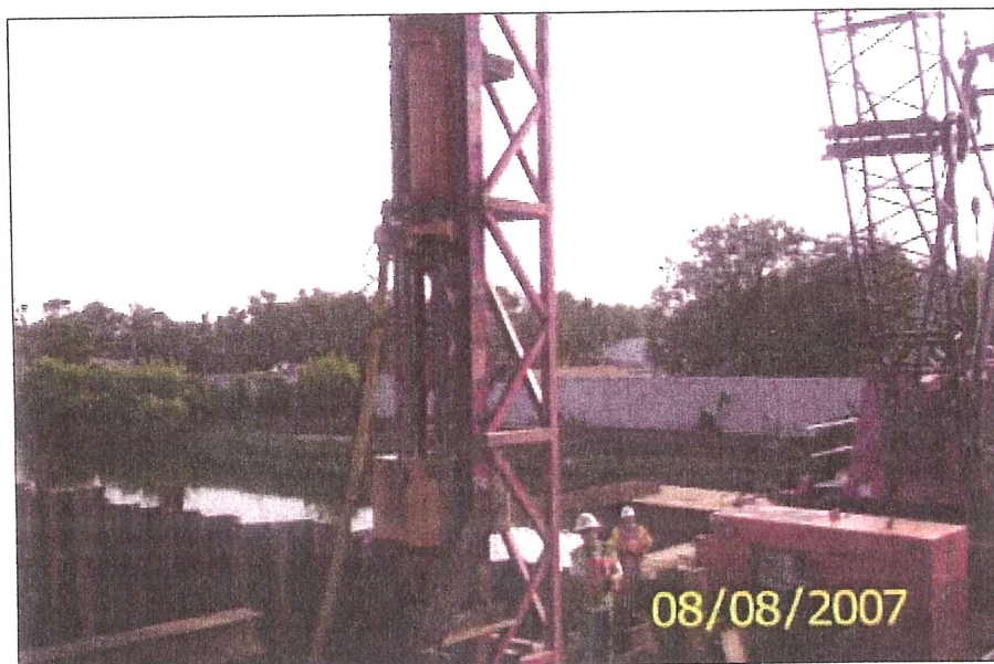
Figure 3.3 – H-Pile Driving Hammer in Swinging Leads
