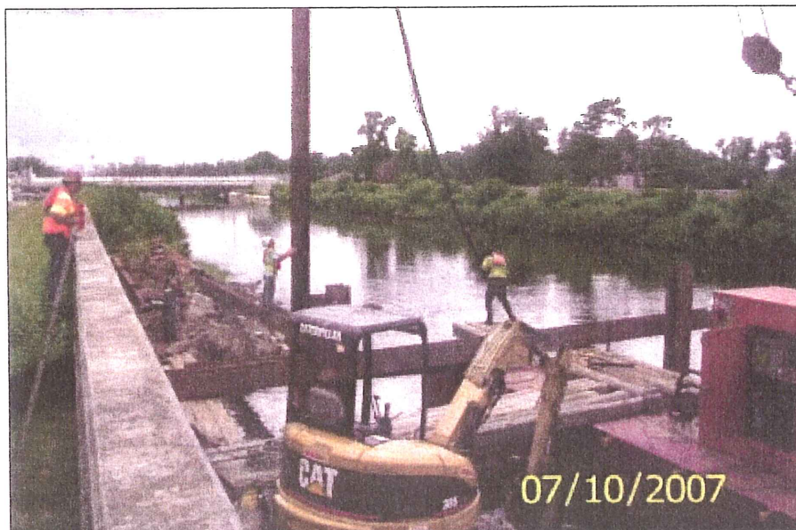
Figure 3.1 – Establishing Sheetpile Template
