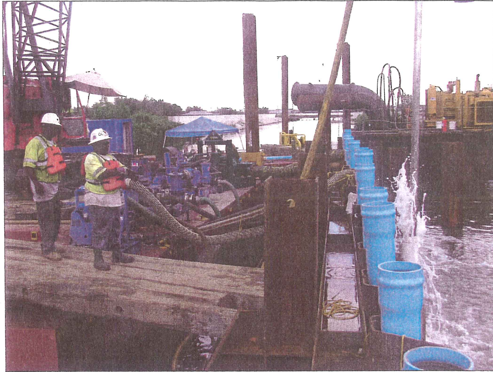
Figure 3.10 – Cleaning Each Slotted Pipe by Water Jetting.
