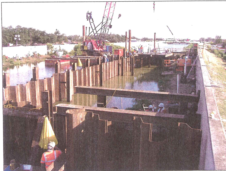
Figure 3.5 – Almost Completed Cofferdam
