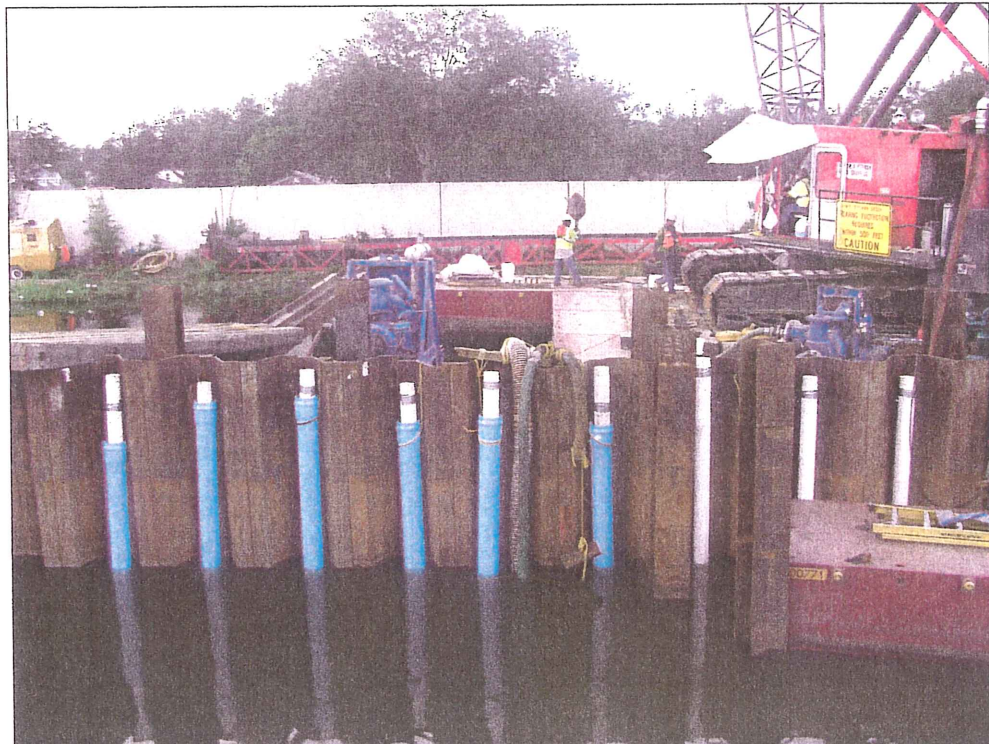
Figure 3.9 – Partially Completed Array of Slotted Pipes.
