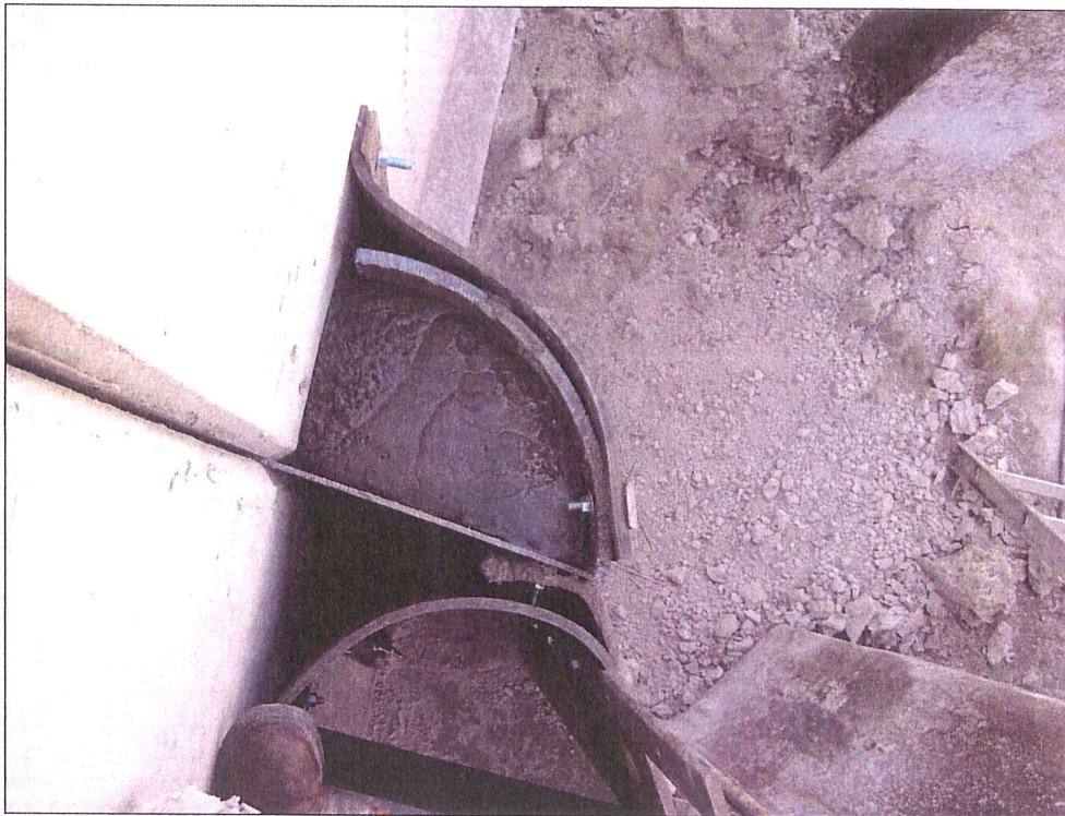
Figure 2.9 – Connection Between Cofferdam and I-Wall
