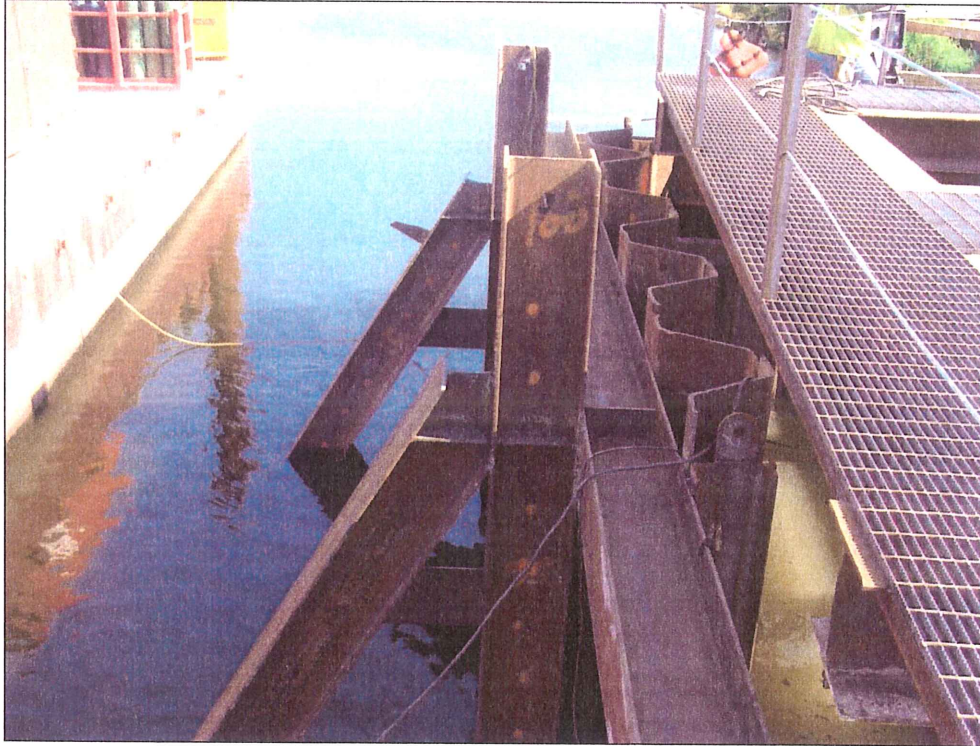
Figure 2.8 – Pile Bent and Waler
