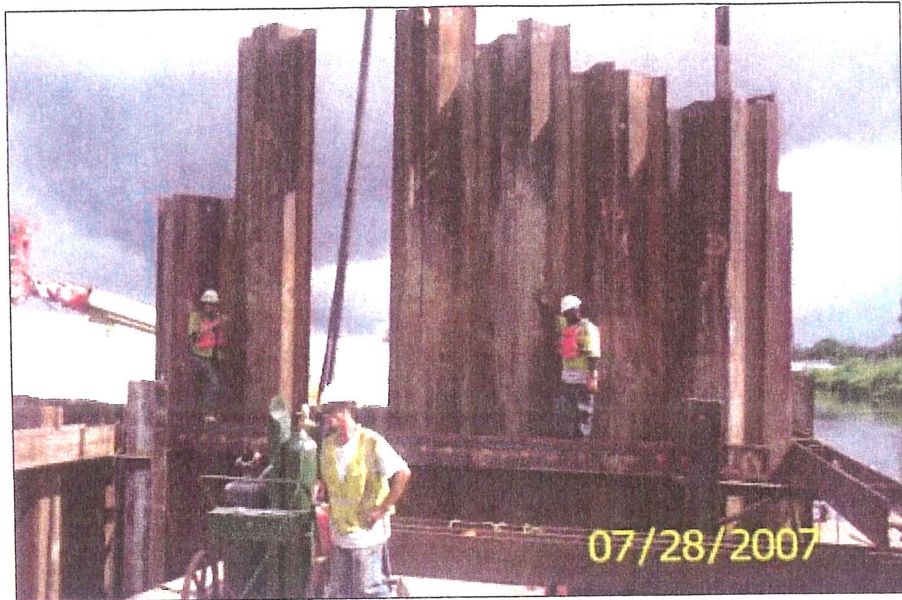
Figure 3.2 – Sheetpile Cofferdam Underway
