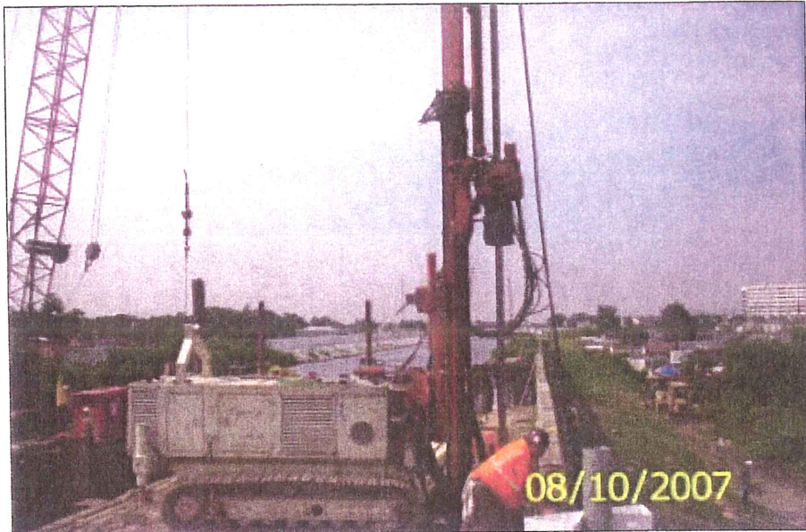
Figure 3.4 – Jet Grouting Operation
