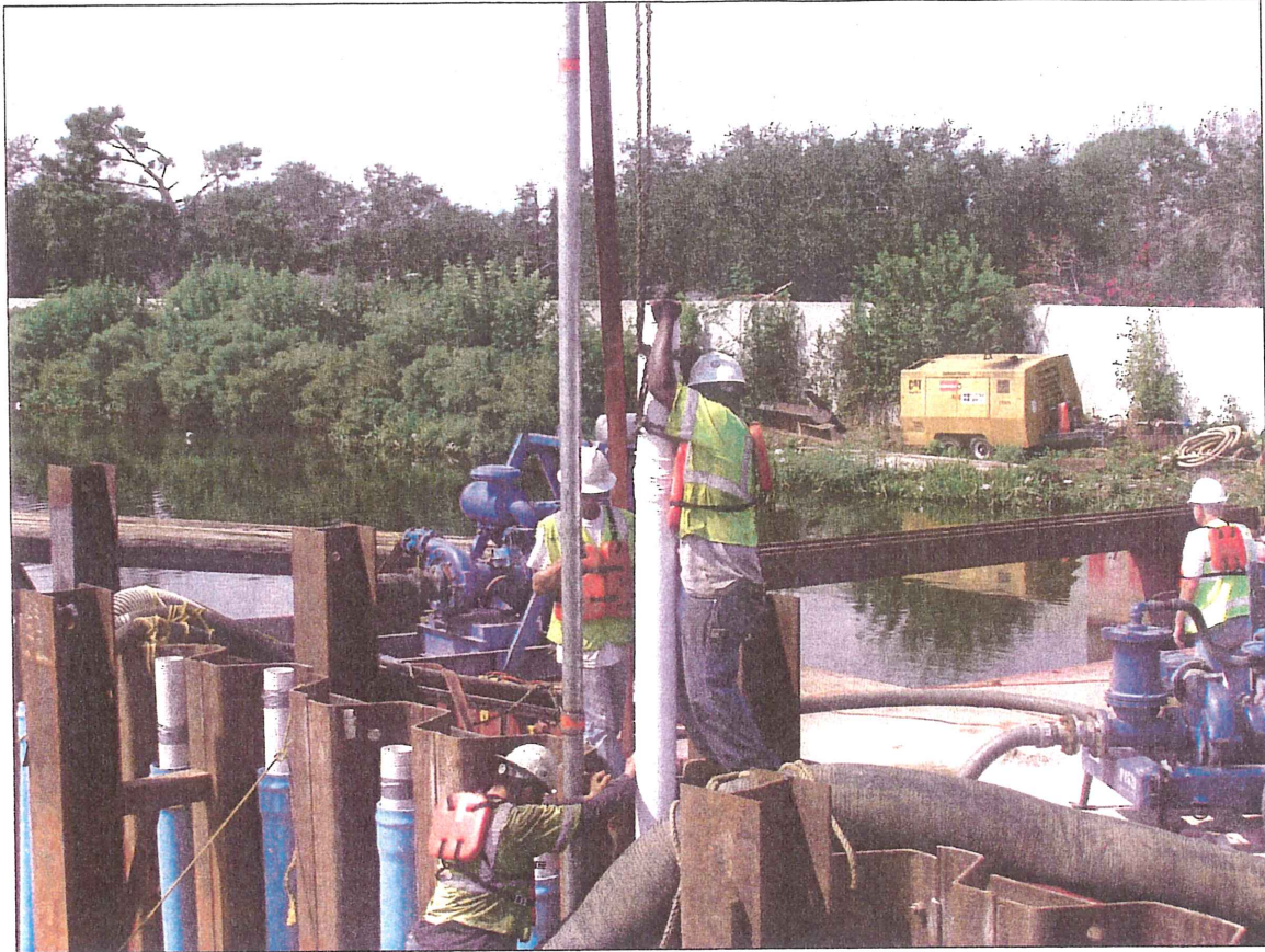
Figure 3.7 – Slotted Pipe Installation Using Jetting Techniques
